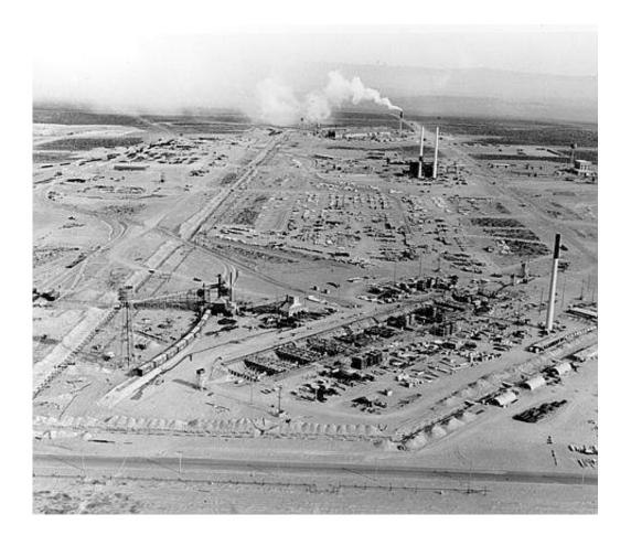
An early picture of the Hanford Site in eastern Washington State. By October 1944, the first plutonium reprocessing facility (T Plant) began operating (in background). U Plant (in the foreground) was under construction in the mid-1940s. Credit: Hanford Site Archives
