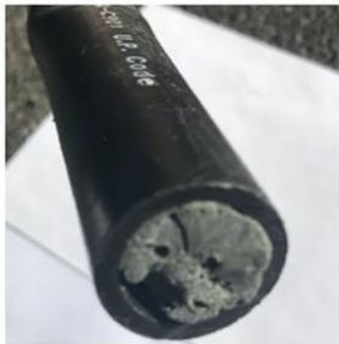
Melted and rehardened plastic inside pipe w/ different color
