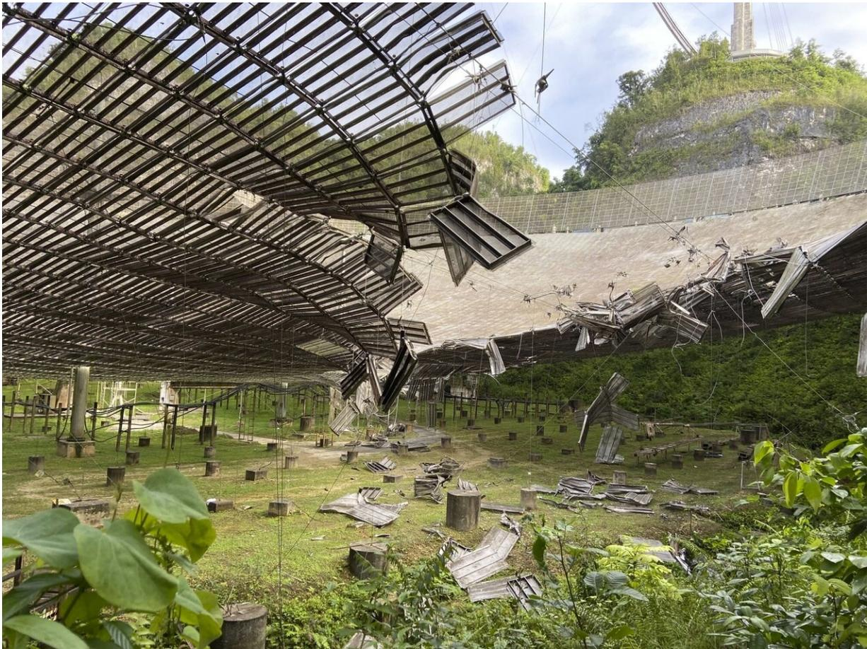
This photo provided by the Arecibo Observatory, shows the damage done by a broken cable that supported a metal platform, creating a 100-foot (30-meter) gash to the radio telescope's reflector dish in Arecibo, Puerto Rico, Tuesday, Aug. 11, 2020. The University of Central Florida that manages the National Science Foundation facility said eight panels in the dome also were damaged and the platform used to access the dome is now twisted. (Arecibo Observatory via
