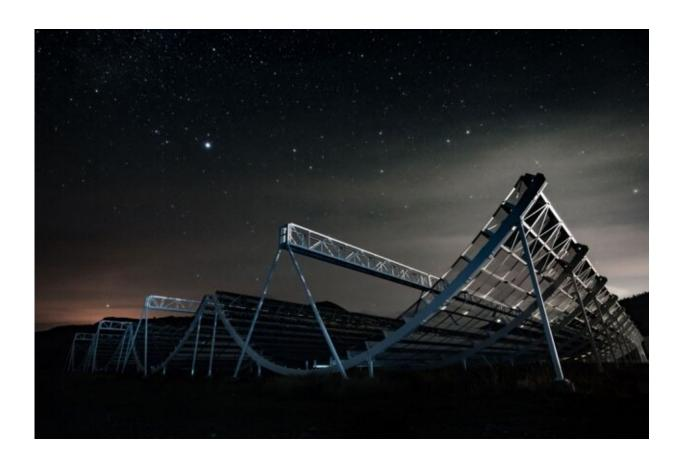
CHIME, pictured here, consists of four large antennas, each about the size and shape of a snowboarding half-pipe, and is designed with no moving parts. Rather than swiveling to focus on different parts of the sky, CHIME stares fixedly at the entire sky, looking for fast radio burst sources across the universe. Credit: CHIME Collaboration
