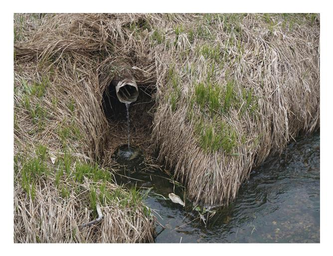
Tile drainage pipes are installed in some fields to help prevent muddy or flooded soil. This tile carries water to a nearby stream. Credit: John Schutte
