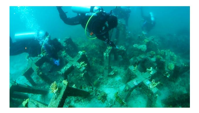
An artificial concrete reef to provide support for unstable coral fragments underwater is installed by Accenture, Intel and Sulubaaï Environmental Foundation in the coral reef surrounding Pangatalan Island in the Philippines. Credit: Accenture
