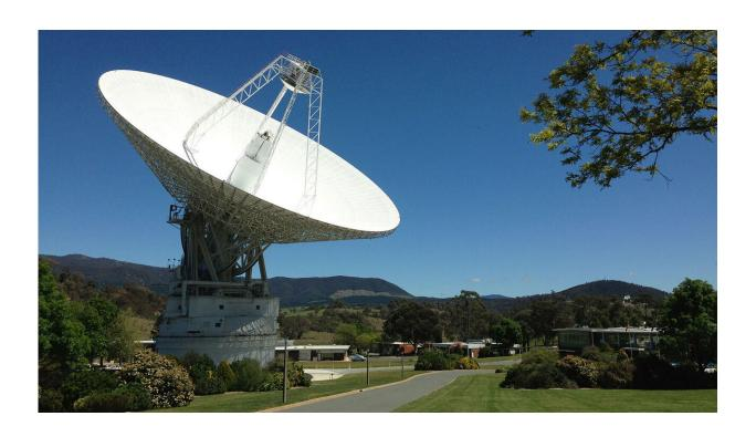
DSS43 is a 70-meter-wide (230-feet-wide) radio antenna at the Deep Space Network's Canberra facility in Australia. It is the only antenna that can send commands to the Voyager 2 spacecraft. Credit: NASA/Canberra Deep Space Communication Complex
