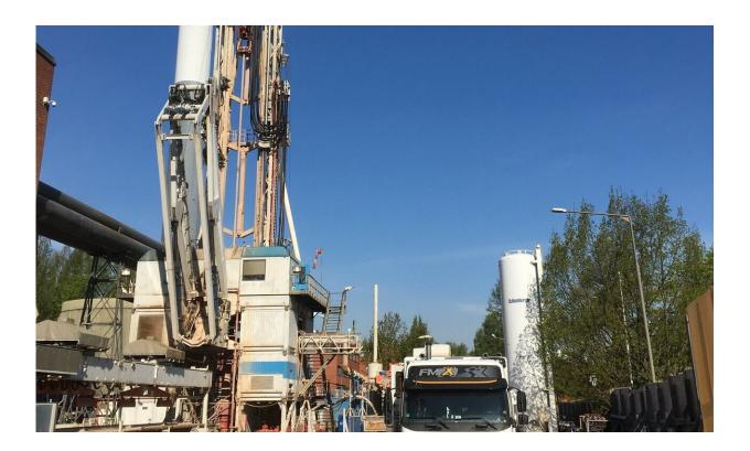
Drilling rig of the geothermal project in Helsinki, Finland. The project aims to supply the university campus with heat from a depth of more than 6 kilometres Credit: G. Dresen
