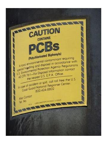
PCB warning label affixed to a railroad signal power supply transformer dating from the 1930's at CP-SLOPE interlocking, west of Altoona, PA on the Norfolk Southern Pittsburgh Line. Credit: Sturmovik/Wikipedia
