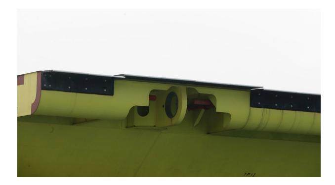
A detail of a hinge of a barrier, part of a plan to protect the city of Venice from flooding, floats on a barge, in Venice, Italy, Friday, Nov. 29, 2019. The barrier system is made up of 78 giant flood gates, each 20 meters long and the gates are attached by hinges to giant cement blocks placed on the seabed along the three openings from the sea into the lagoon, Malamocco, Chioggia and the Lido. (AP Photo/Antonio Calanni)
