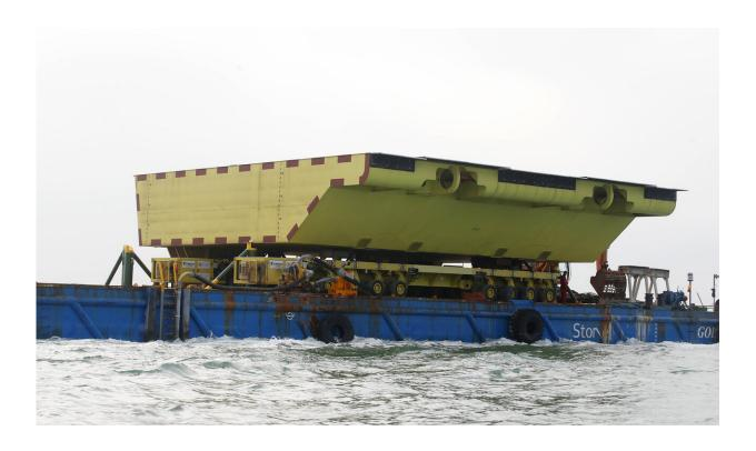
A yellow barrier, part of a plan to protect the city of Venice from flooding, floats on a barge, in Venice, Italy, Friday, Nov. 29, 2019. Central to the plan to protect Venice, some, or all, of the 78 barriers will one day be raised when the sea rises more than 110 centimeters to prevent damaging high tides from pushing into the lagoon city, a UNESCO heritage site built picturesquely but somewhat precariously among more than 120 islands. (AP Photo/Antonio Calanni)
