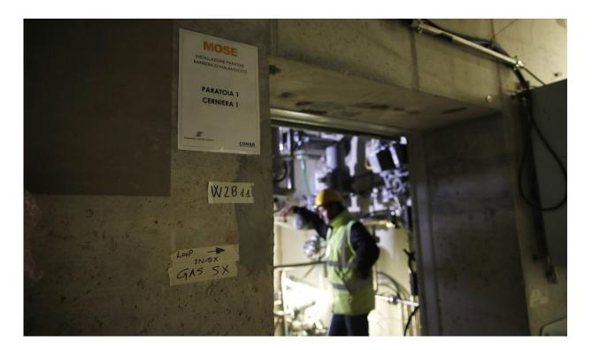
A worker walks in an undersea tunnel part of a plan to protect the city of Venice from flooding, in Venice, Italy, Friday, Nov. 29, 2019. The barrier system is made up of 78 giant flood gates, each 20 meters long which are attached by hinges to giant cement blocks placed on the seabed along the three openings from the sea into the lagoon, Malamocco, Chioggia and the Lido. (AP Photo/Antonio Calanni)
