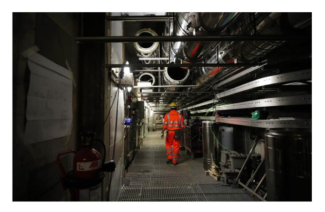
A worker walks in an undersea tunnel part of a plan to protect the city of Venice from flooding, in Venice, Italy, Friday, Nov. 29, 2019. The barrier system is made up of 78 giant flood gates, each 20 meters long which are attached by hinges to giant cement blocks placed on the seabed along the three openings from the sea into the lagoon, Malamocco, Chioggia and the Lido. (AP Photo/Antonio Calanni)
