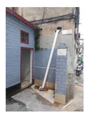
Self-installed flush toilets like this one in Shanghai often just empty into rainwater drains. Credit: Deljana Iossifova, Author provided
