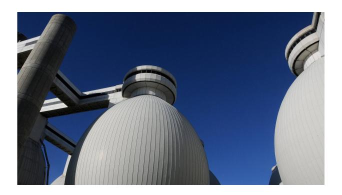
Anaerobic digesters, like those pictured here, can be used to convert sewage sludge and fatty waste into natural gas. Photo credit: Rachel Schowalter. Shared by the Massachusetts Clean Energy Center under a Creative Commons license.
