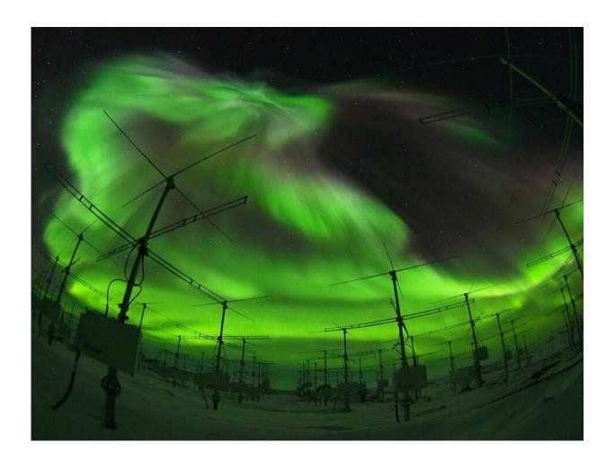
The Program of the Antarctic SyowaMesosphere-Stratosphere-Troposphere/Incoherent Scatter radar (PANSYradar) consisting of an active phased array of 1045 Yagi antennas. Credit: Taishi Hashimoto (NIPR)
