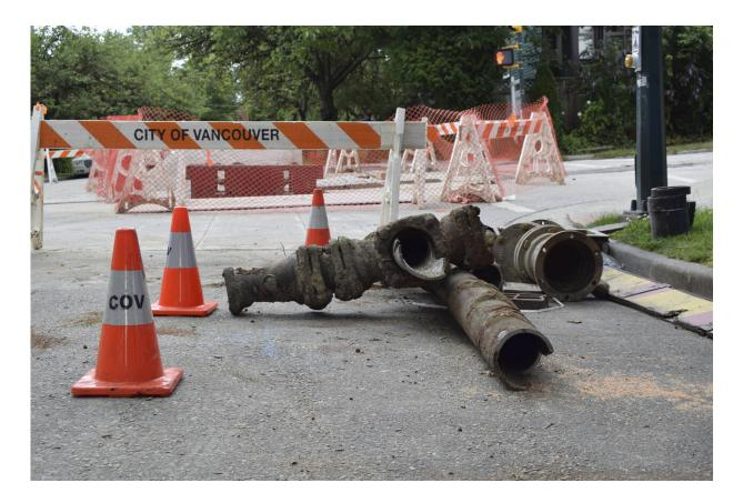
Unearthed pipes lie on Vancouver's East 12th Avenue, which is undergoing construction to replace a water main on July 14, 2019. According to the City of Vancouver, the existing water main is predicted to be over 100 years old, having been installed between 1906 and 1909. In Canada, where provinces—not the federal government—set water safety rules, the main source of lead in drinking water is antiquated pipes. (Mackenzie Lad/Institute for Investigative Journalism/Concordia University via AP)
