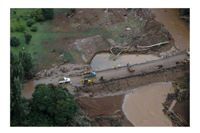
This March 14, 2006, file photo, shows damage after a dam burst near Kilauea, on the Hawaiian island of Kauai. An earthen wall of the Kaloko Reservoir collapsed during heavy rains and sent a wave of water and mud rushing down a hillside. Seven people were killed on Bruce Fehring's property, including his daughter, son-in-law and grandson. (AP Photo/Casey Riemer, File)
