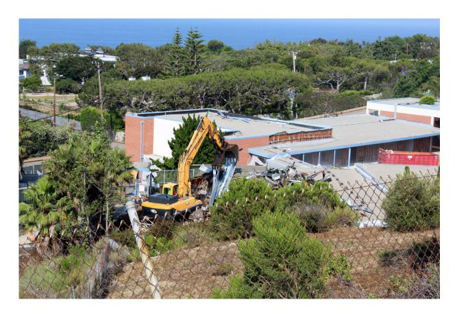
This July 5, 2017, image provided by Malibu Surfside News shows the demolition of the former Malibu Middle School in California. The school was torn down after testing found high levels of PCBs, which were used in some caulk, floor adhesive and in fluorescent light ballasts until the chemicals were banned in the late 1970s over fears that they could cause cancer. (Barbara Burke/Malibu Surfside News via AP)
