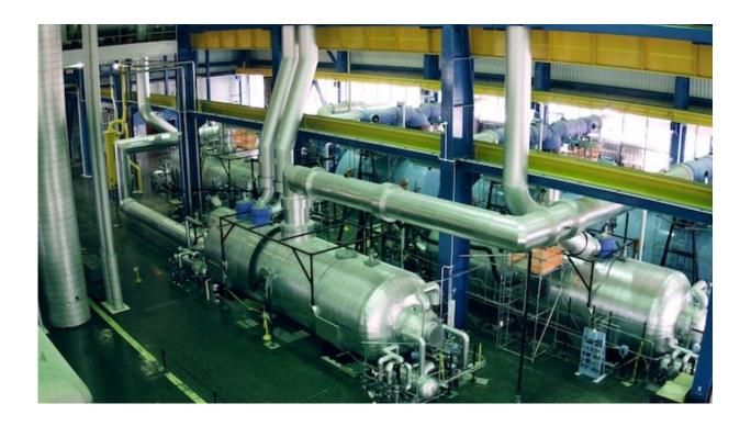
Nuclear power plants contain miles of pipes of different sizes. Shown is the turbine floor with new reheaters and secondary side piping at Unit 2, Watts Bar Nuclear Power Plant, 2012. Credit: Tennessee Valley Authority
