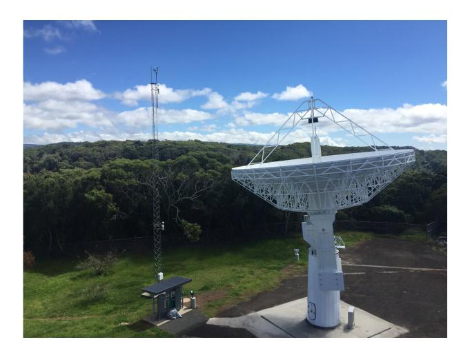
Banner Image: The next-generation radio telescope at Kokee Park in Hawaii, built as part of the Space Geodesy Project, is smaller and faster than older VLBI technology, making it more adaptable to atmospheric conditions. Credit: NASA
