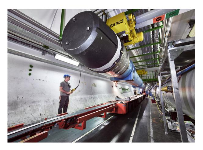
Replacement of one of the LHC superconducting dipole magnets during the accelerator consolidation campaign. Credit: Maximilien Brice and Julien Ordan/CERN
