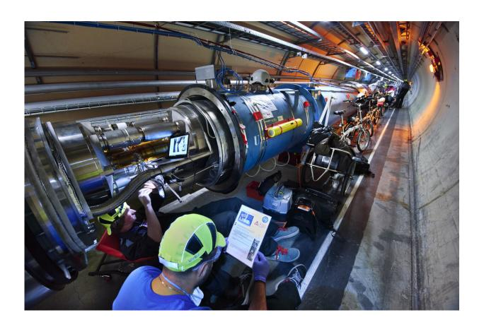
Two members of the LHC consolidation team inspect and clean a diode enclosure of the dipole magnets before improving the electrical isolation. Credit: Maximilien Brice and Julien Ordan/CERN
