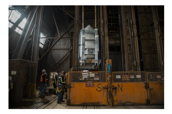
Crews at the Sanford Underground Research Laboratory in Lead, South Dakota, begin to lower the LUX-ZEPLIN central detector. Its nearly mile-long descent down an elevator shaft, and its delivery to a research cavern where it will hunt
