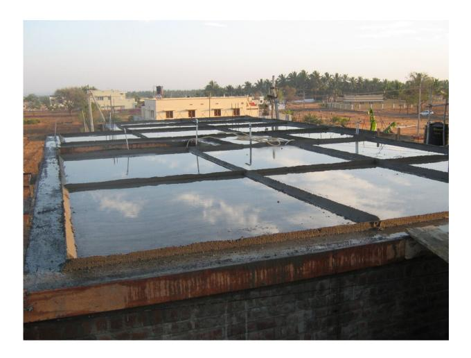
For concrete to properly harden, or cure, a consistent level of moisture must be present throughout the material as it sets. To do this contractors will spray it with water or create pools on top. Credit: Drexel University
