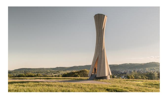
Urbach Tower, a 14 m tall building demonstrator with high curvature CLT components produced using self-shapping manufacturing technology. Credit: ICD/ITKE University of Stuttgart
