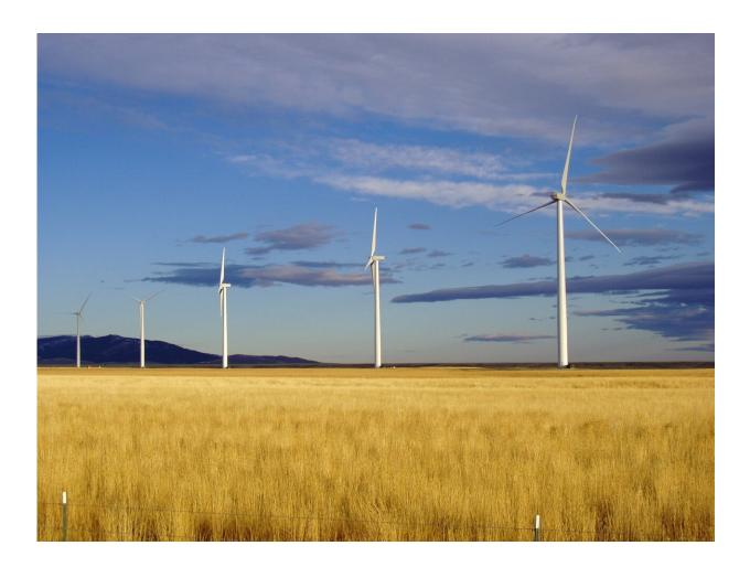
The Judith Gap Wind Energy Center in Montana is comprised of 90 GE 1.5-MW turbines, for a total capacity of 135 MW. Credit: Invenergy LLC, NREL.
