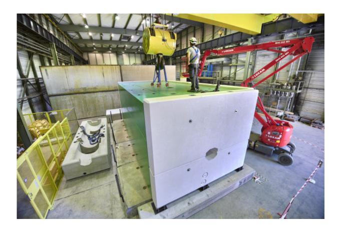
The beam dump's shielding being assembled. Credit: Maximilien Brice/CERN
