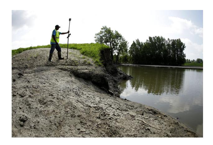
In this Tuesday, Aug. 6, 2019 photo, U.S. Army Corps of Engineers worker Ron Allen uses a GPS tool to survey the extent of damage where a levee failed along the Missouri River near Saline City, Mo. Efforts to fight rising waters may turn out to be only down payments on what is shaping up as a long-term battle against floods, which are forecast to become more frequent and destructive as global temperatures rise. (AP Photo/Charlie Riedel)
