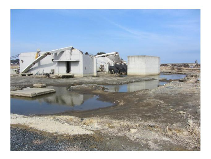
A scene following the 2011 Heisei Tsunami in Idagawa, Fukushima, Japan, showing destruction of a reinforced-concrete structure and severe scour surrounding the structure. Credit: OSU College of Engineering
