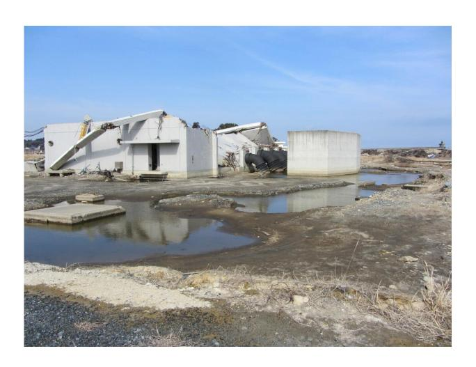
A scene following the 2011 Heisei Tsunami in Idagawa, Fukushima, Japan, showing destruction of a reinforced-concrete structure and severe scour surrounding the structure. Credit: OSU College of Engineering
