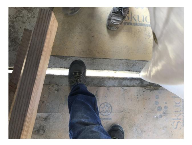
In this July 22, 2019, photo, gaps are being built into Oregon State University's Marine Studies Building to make it earthquake resistant in Newport, Ore. Construction workers in this Oregon coastal town are erecting a school building, right in the path of a future tsunami that experts say will be generated by a huge offshore earthquake that is certain to occur sooner or later. (AP Photo/Andrew Selsky)
