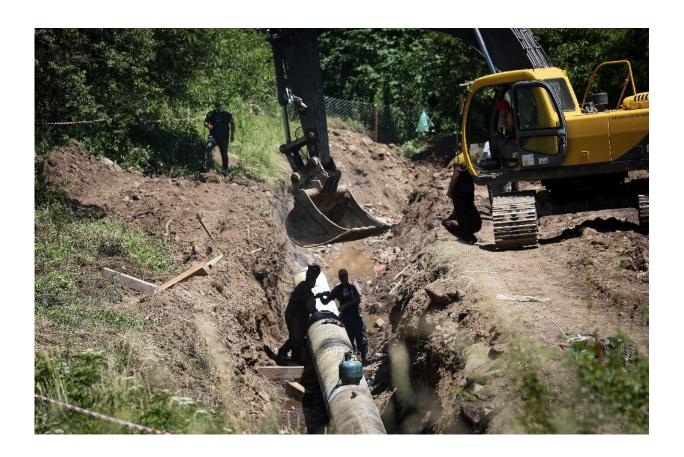
Pipes will divert up to 90 percent of the water from Rakita's river to an energygenerating turbine
