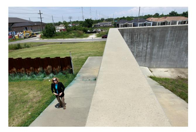
In this May 15, 2012, file photo, Sandy Rosenthal, founder and director of levees.org, stands near a section of the old levee wall, I-wall made of sheet piling, left, and the new levee wall, t-walls with reinforced concrete, at one of the breach sites from Hurricane Katrina, in the Lower 9th Ward in New Orleans. "The models for Hurricane Katrina were all wrong," Rosenthal said. "We don't care what the model says. The model is an educated guess. That's all it is." (AP Photo/Gerald Herbert, File)
