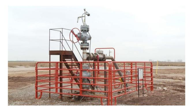
Oil and gas production requires the disposal of wastewater, which is injected into rock formations far underground through wells such as this. To minimize earthquake hazards from this process, an ASU-led team has created a new model for forecasting induced seismicity from wastewater injection. Credit: KFOR-TV, Oklahoma City
