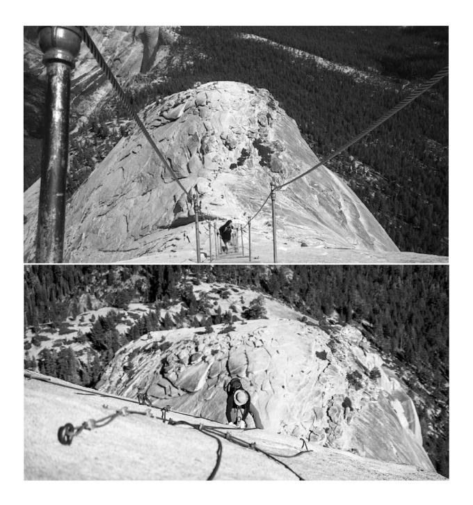
Cables in the upright position (May-September) and down position (off-season). When upright, the cables literally create handrails with wooden foot supports. In
