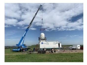
KITcube mobile measurement facility: with the help of a truck crane, the precipitation radar is installed at Müglitztal/Saxony. Credit: Dr. Andreas Wieser, KIT
