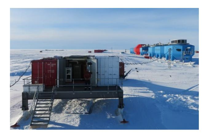
The Automation platform at Halley Research Station provides power to science kit from a micro-turbine (main station in background). Credit: British Antarctic Survey
