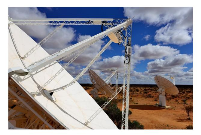
ASKAP's dish antennas feature a novel phased array feed (PAF) receiver, that enable a massive 30 square degree wide-field view on the sky. Credit: CSIRO/Dragonfly Media
