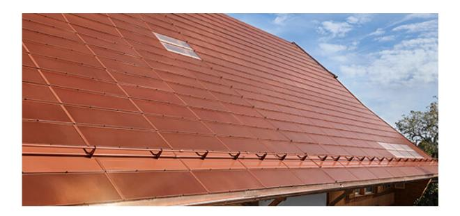
Renovation project with active terracotta tiles based on monocrystalline silicon cells. This farmhouse in Ecuvillens (canton of Fribourg) is situated in a conservation area in which roof-mounted photovoltaic modules are prohibited. Credit: Patrick Heinstein
