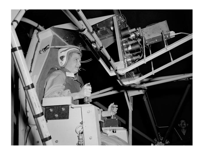
In this 1960 photo made available by NASA, Jerrie Cobb prepares to operate the Multi-Axis Space Test Inertia Facility (MASTIF) at the Lewis Research Center in Ohio. The three-axis rig was developed to train Project Mercury pilots in bringing a spinning spacecraft under control. The two controllers in Cobb's hands activated small nitrogen gas thrusters that were used to bring the MASTIF under control. She was one of several female pilots who underwent the skill and
