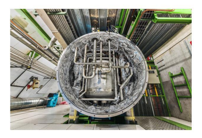
One of the LHC cold boxes, located in an underground cavern at point 4 of the ring. Liquid helium is stabilised and stored in a tank at a temperature of approximately 4.5 K. Credit: CERN
