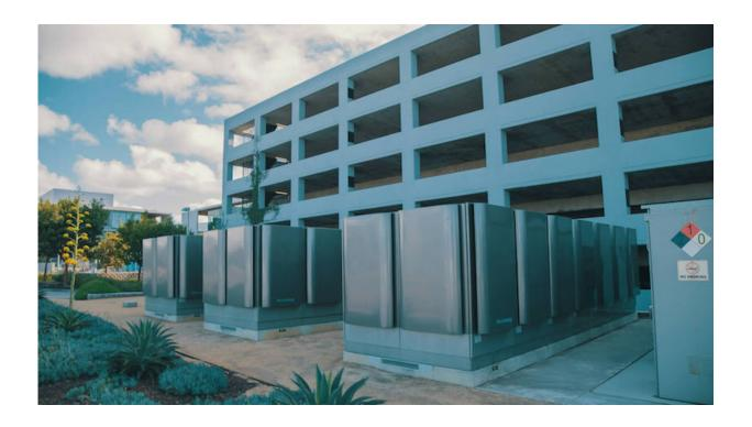
Solid oxide fuel cells can be used in a variety of applications, including efficiently generating primary or emergency backup power for buildings. A group of Bloom Energy Servers generates power using solid oxide fuel cells. Credit: Bloom Energy
