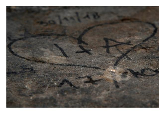
The laser evaporates the graffiti without damaging the stone underneath
