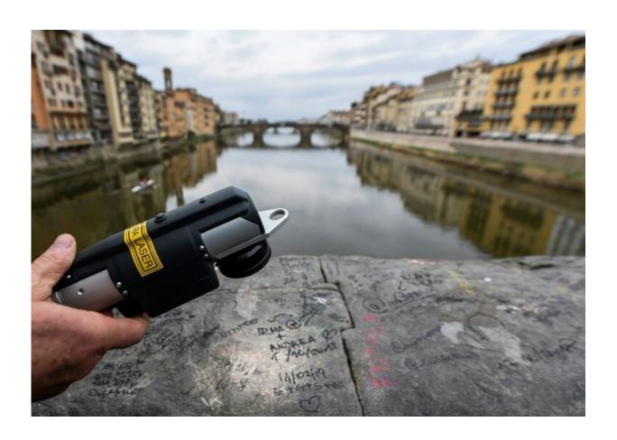
A latest-generation infrared wand is being used to remove graffiti spoiling the city of Florence
