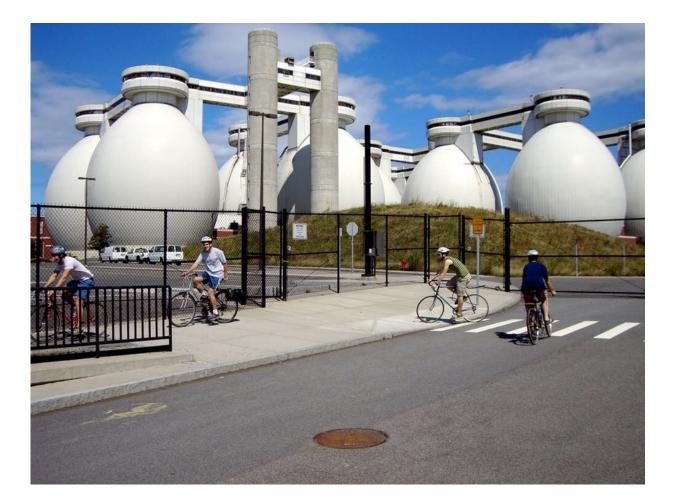
Inside these anaerobic 'egg' digesters at the Deer Island Treatment Plant on Boston Harbor, microbes break down sewage sludge and scum into methane gas, carbon dioxide, water and organic solids that are processed into fertilizer. Credit: <u>Frank Hebbert/Wikimedia</u>, <u>CC BY</u>
