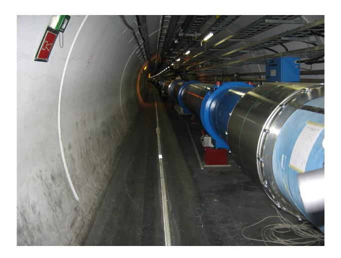
Large Hadron Collider dipole magnets. Credit: CERN
