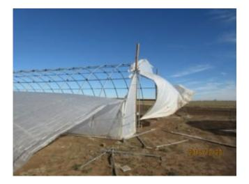
Within weeks of completion of the first high tunnel in 2015, severe straight-line winds nearly blew one completely out of the ground. Credit: Texas A&M AgriLife photo by Jimmy Gray
