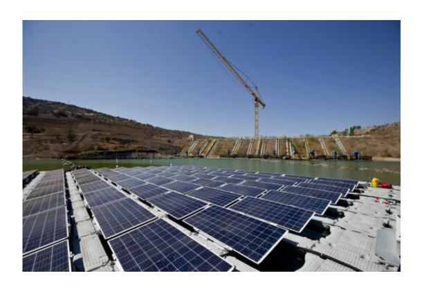
An island of solar panels floats in a pond at the Los Bronces mining plant, about 65 kilometers (approximately 40 miles) from Santiago, Chile, Thursday, March 14, 2019. The island of solar panels could give purpose to mine refuse in Chile by using them to generate clean energy and reduce water evaporation.(AP Photo / Esteban Felix)
