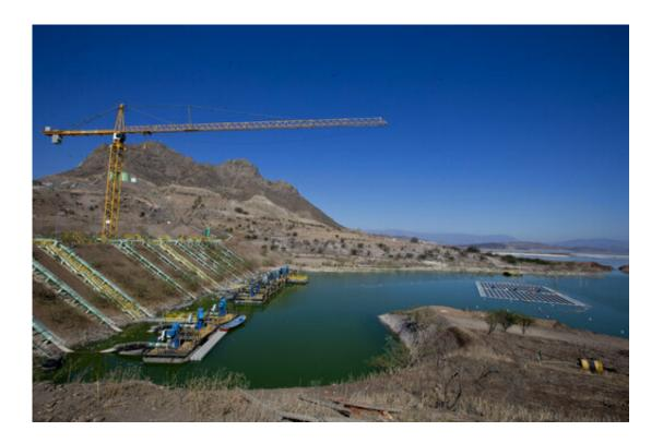
An island of solar panels floats in a pond at the Los Bronces mining plant, about 65 kilometers (approximately 40 miles) from Santiago, Chile, Thursday, March 14, 2019. The array floats in the middle of a pond that is used to contain the refuse from mining, known as tailings, and it is expected that the island's shadow will lower the water temperature and reduce evaporation by 80 percent. (AP Photo/Esteban Felix)
