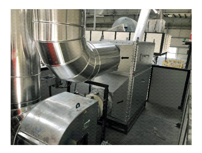
Heat pipe heat exchanger. Credit: Brunel University
