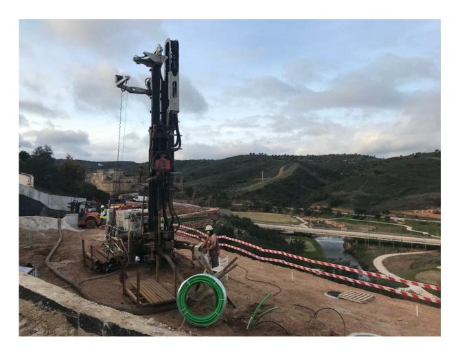
Drilling process of a real-world geothermal borehole at an ongoing construction site in Portugal. Credit: Daniel Muñoz of Sacyr Industrial.
