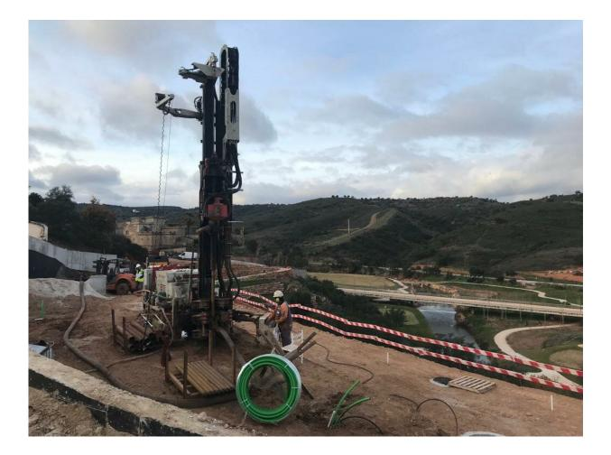
Drilling process of a real-world geothermal borehole at an ongoing construction site in Portugal. Credit: Daniel Muñoz of Sacyr Industrial.
