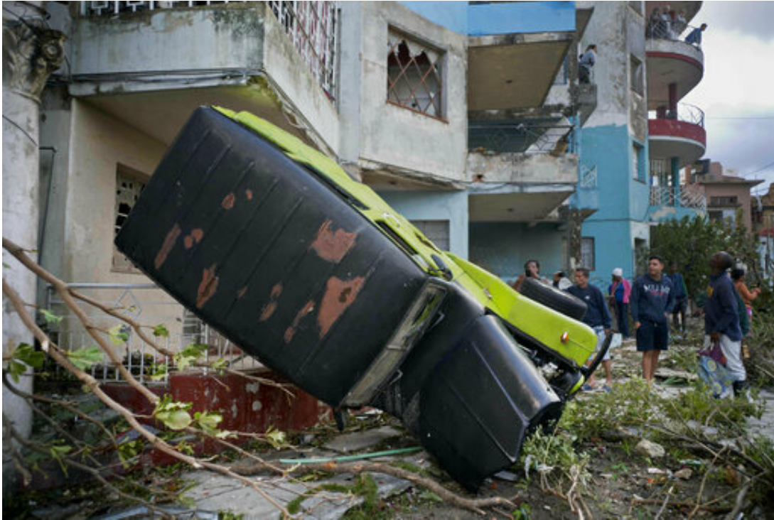
A truck is toppled against a home after a tornado in Havana, Cuba, Monday, Jan. 28, 2019. A tornado and pounding rains smashed into the eastern part of Cuba's capital overnight, toppling trees, bending power poles and flinging shards of metal roofing through the air as the storm cut a path of destruction across eastern Havana. (AP Photo/Ramon Espinosa)
