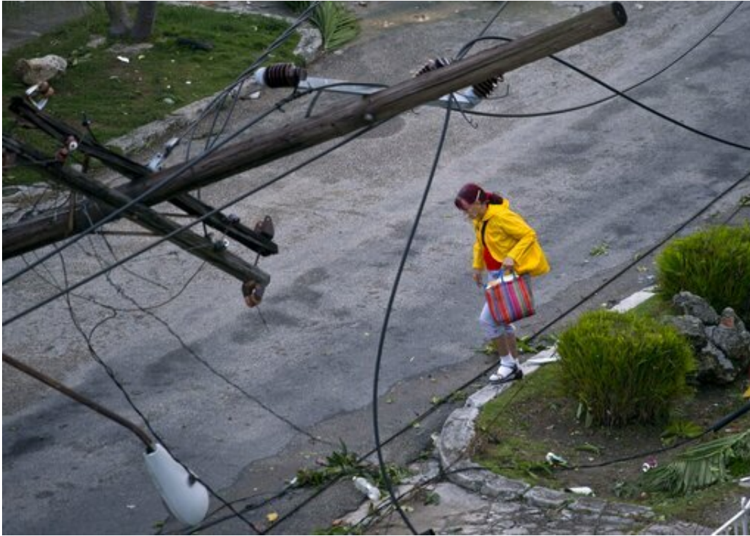
A woman walks under a lamp post toppled by a tornado in Havana, Cuba, Monday, Jan. 28, 2019. A tornado and pounding rains smashed into the eastern part of Cuba's capital overnight, toppling trees, bending power poles and flinging shards of metal roofing through the air as the storm cut a path of destruction across eastern Havana. (AP Photo/Ramon Espinosa)
