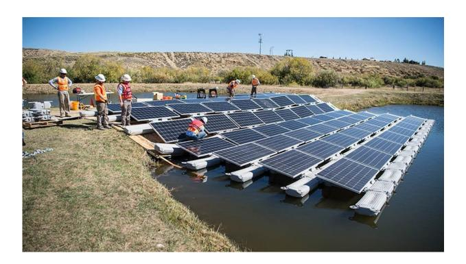
Floating PV being installed in Walden, Colorado. Credit: Dennnis Schroeder/NREL
