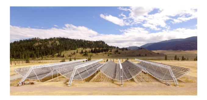
The CHIME telescope incorporates four 100-metre long U-shaped cylinders of metal mesh that resemble snowboard half-pipes, with total area equivalent to five hockey rinks. CHIME reconstructs the image of the overhead sky by processing the radio signals recorded by thousands of antennas. Its signal processing system is the largest of any telescope on Earth, allowing it to search huge regions of the sky simultaneously. Credit: CHIME
