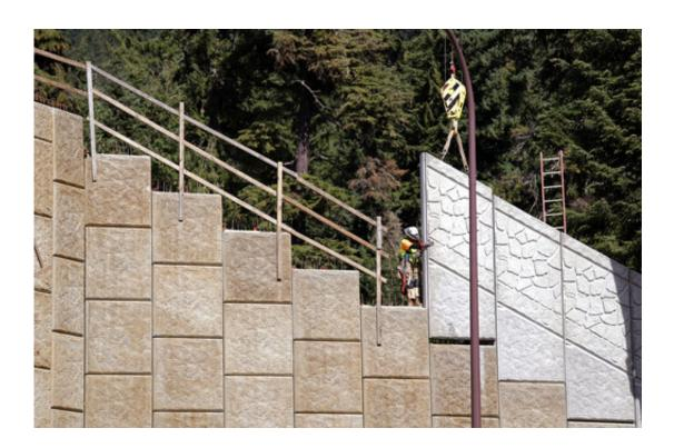
In this photo taken Oct. 4, 2018, a worker helps install tall panels on a wildlife bridge under construction over Interstate 90 on Snoqualmie Pass, Wash. The stretch of highway crossing the Cascade Mountains cuts through old growth forest and wetlands, creating a dangerous border for wildlife everything from an elk down to a small salamander. The new crossing gives animals in these mountains a safer option for crossing the road: They'll be able to go above it. (AP Photo/Elaine Thompson)
