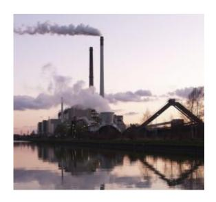
A coal power plant in Datteln, Germany, that transforms chemical energy into 36%-48% electricity and the remaining 52%-64% into waste heat. Image credit: Arnold Paul. Wikimedia Commons.
